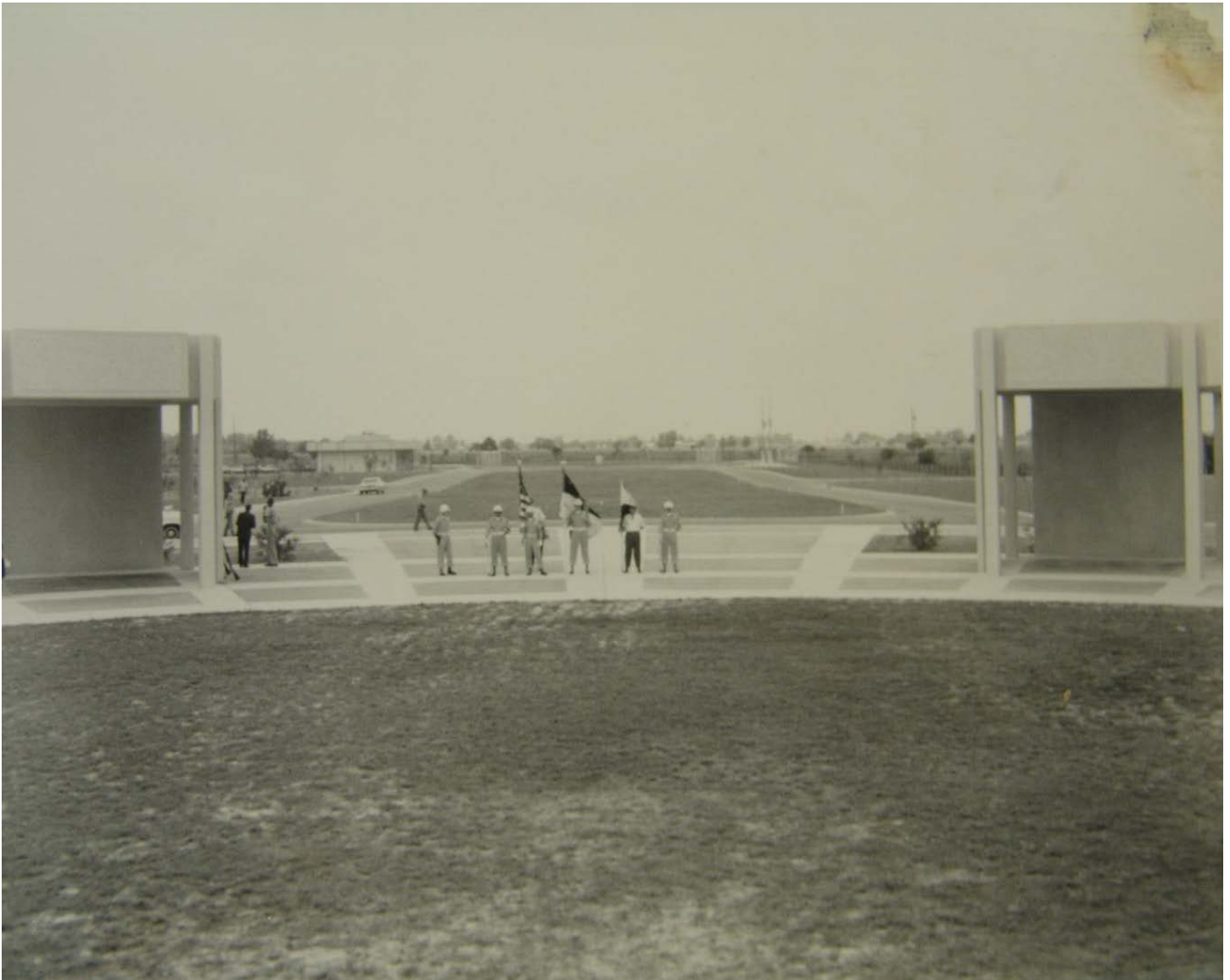
Figure 1. View from hemicycle toward the original cemetery entry flanked by the administration building (left) and flagstaffs (right). ca. 1965. Undated photo. Houston National Cemetery Scrapbook, 1964-1967, compiled by Alwin D. Farrior.
