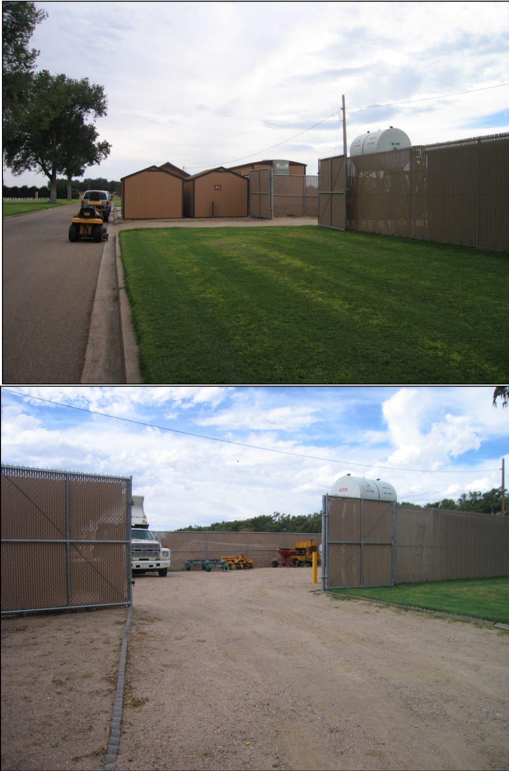
Figure 14. View of Maintenance Yard and Gate 2 opening onto Avenue A in 2005.
