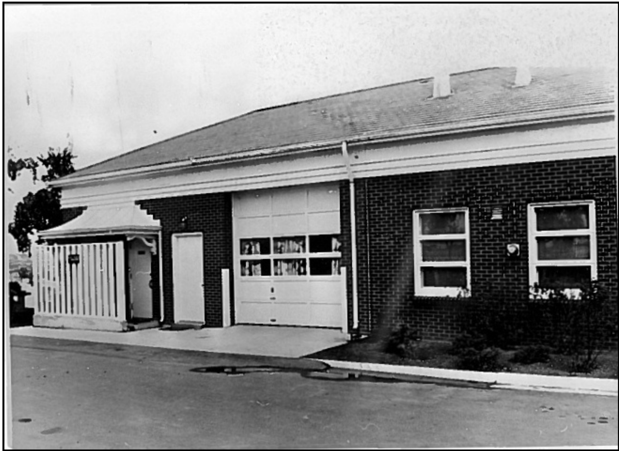
Figure 13: Fort Logan National Cemetery, front of Service Building, west-facing side, 1978 (5DV.11489). Unknown photographer. On file with the Office of Archaeology and Historic Preservation and the VA Historic Preservation Office.
