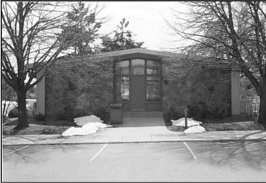
Figure 12: Fort Logan National Cemetery, front of Administration Building/Visitor's Building, 1993 (5DV.9008). Photographer: URS Corp. No longer extant (demolished 2004). On file with the Office of Archaeology and Historic Preservation and the VA Historic Preservation Office.
