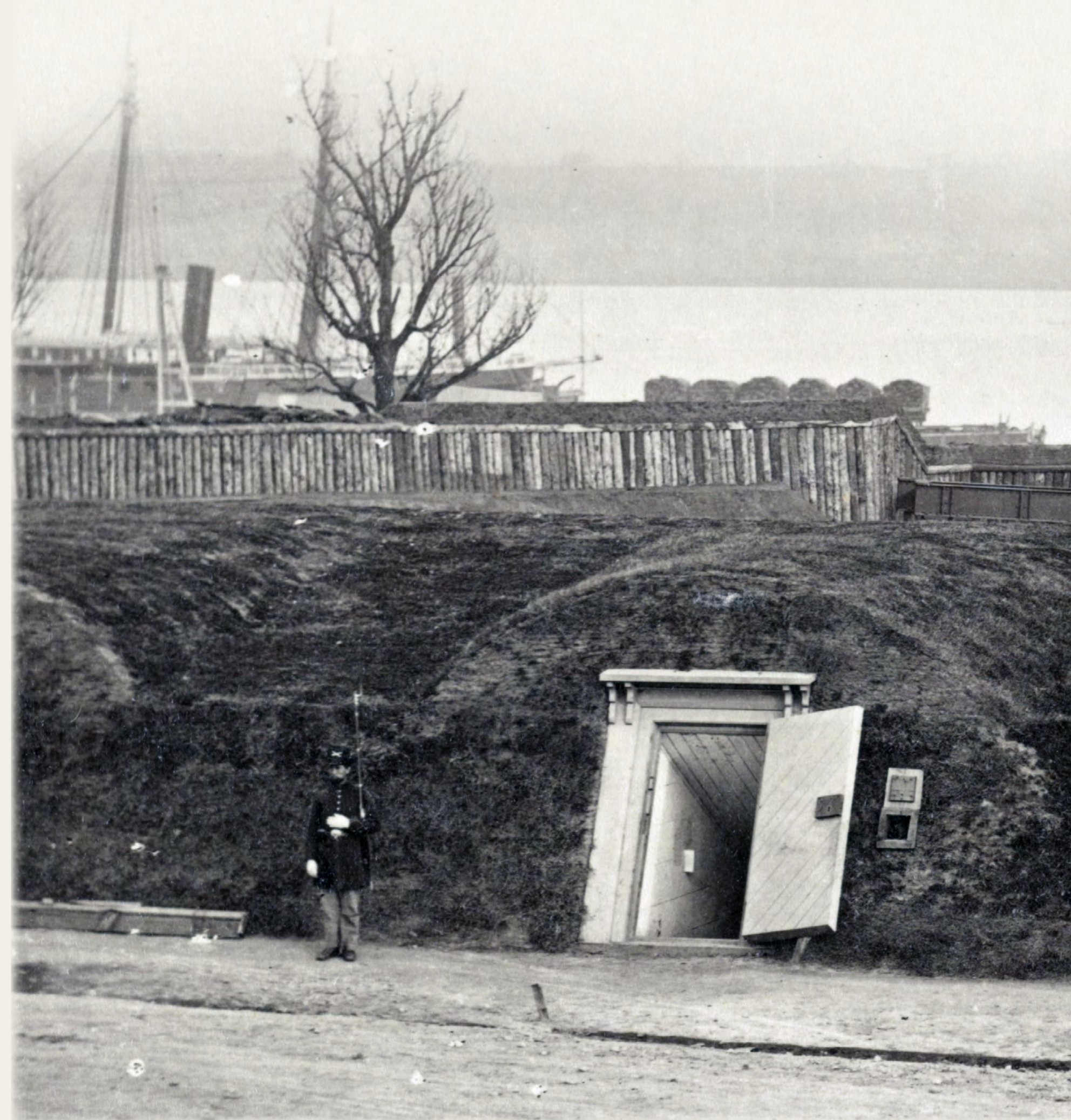
Battery Rogers, Alexandria harbor, was one of ninety-three detached batteries that made up the defenses of Washington, c. 1864. Library of Congress.
