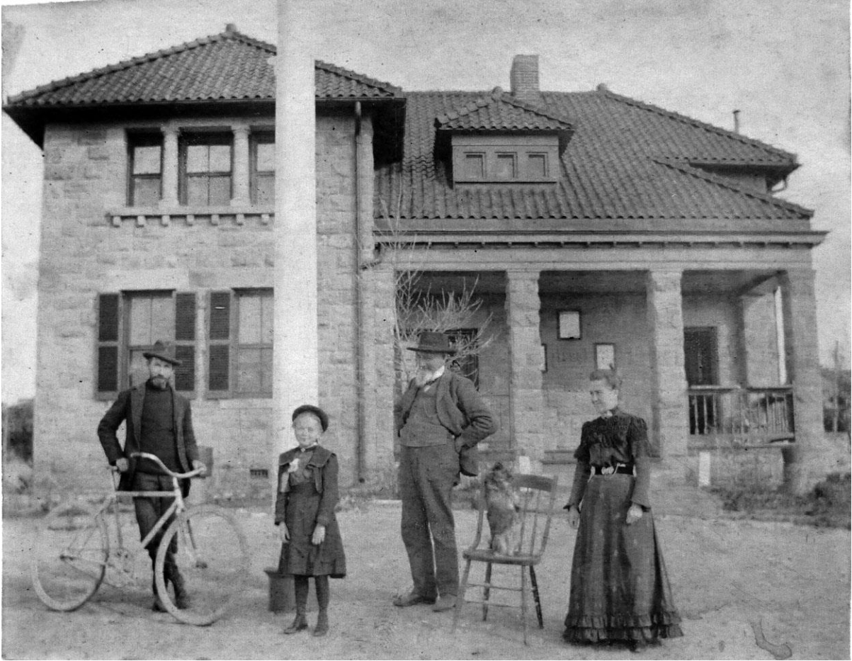
Fig. 14. The stone lodge at Santa Fe, New Mexico, built of local sandstone to an expanded version of the L-plan in 1895. Photograph taken in 1905. National Archives and Records Administration, College Park, Md., Still Picture Branch, RG 92-CA, box 1, folder 17.
