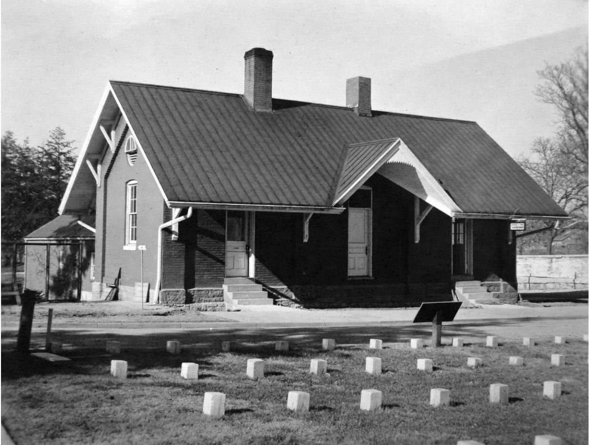
Fig. 5. The 1869 linear-plan brick lodge at Jefferson Barracks National Cemetery, Missouri, designed by Edward Clark, photographed ca. 1935 after being remodeled into an office building and comfort station. The features that led inspector Oscar Mack to call this the "Railway Depot style" are apparent. National Archives and Records Administration, Washington, D.C., Records of the Department of Veterans Affairs, Department of Memorial Affairs, National Cemetery Historical File (Record Group 15/A-1, Entry 25), maintenance ledger pages for Jefferson Barracks.
